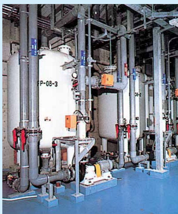
▲Eslon Valves for Aquarium piping.
